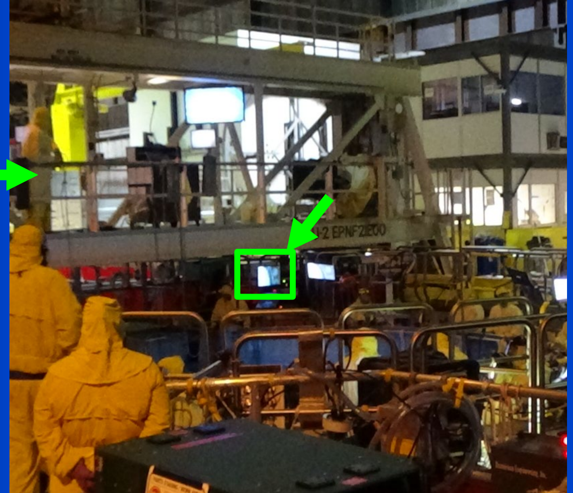
AI Monitor positioned next to Primary Inspection Monitor
